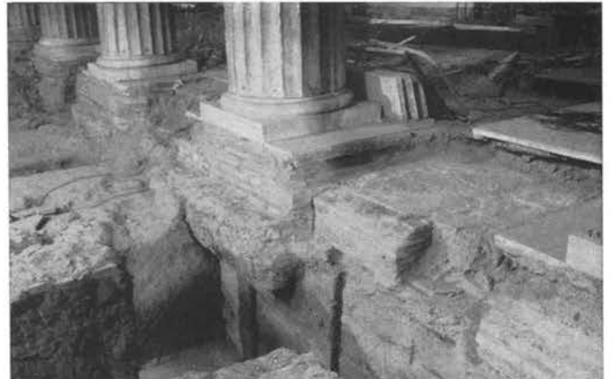
Fig. 163 c . S. Pietro in Vincoli, South colonnade, footing between columns 5, 6 and 7
